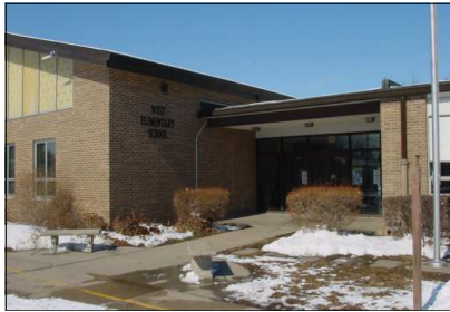
West Elementary School Carlinville, IL
